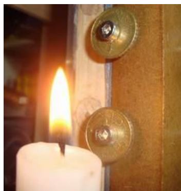
Approximate location of the leak by using a candle
