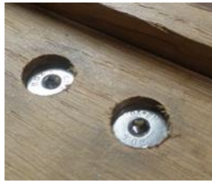
Visible screw heads on the keyframe (they can be hidden with wood filler paste).
